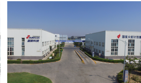
Sunresin, System Engineering Park
