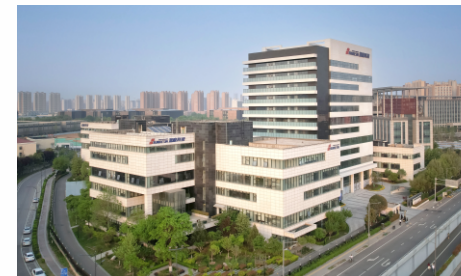
Sunresin Park, Headquarter
