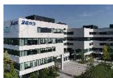
Sunresin Park, Headquarter
